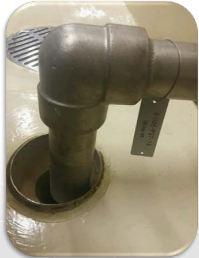
Equipmnet Drain Hole
