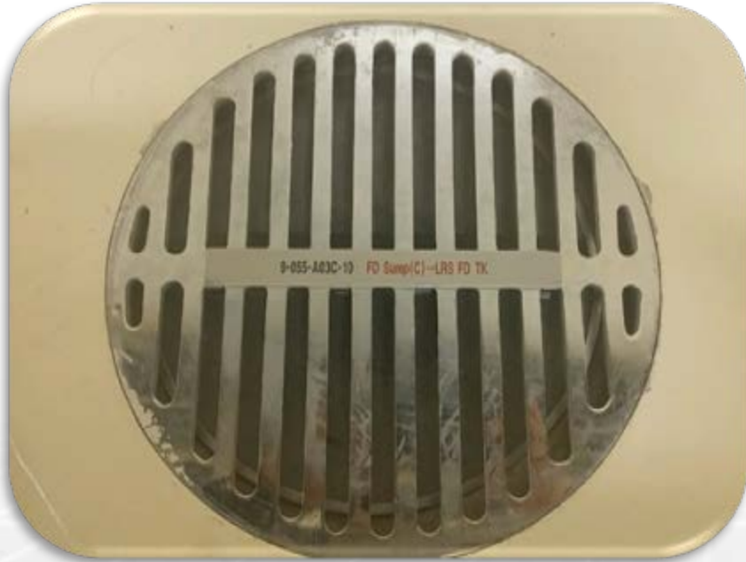
Floor Drain Hole
