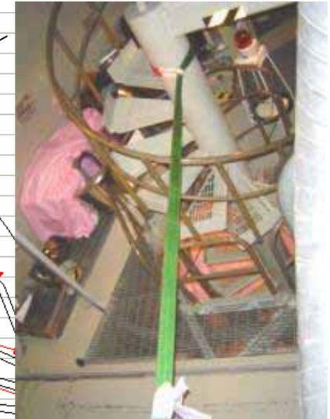
When SRVs disassembling, the lines connected SRVs are needed to be removed. Drawing directions should be determined in advance.
