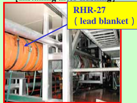
[Installing after flushing]
