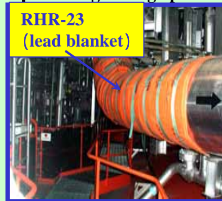
[Installing during operation]
