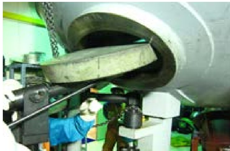
Installation of temporary cover
