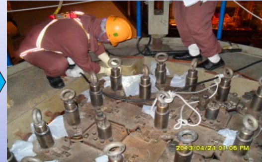
Disassemble Seismic Plate
