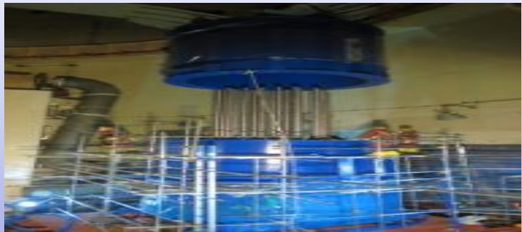
Disassemble Shipping Container
