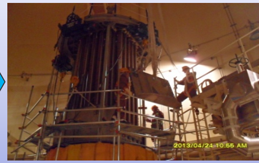
Disassemble Shroud
