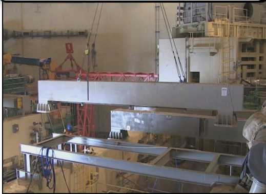
7 Disassembly of the PWR
