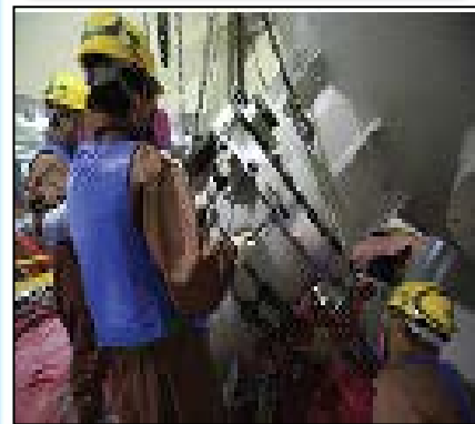
RCS pipes Welding
