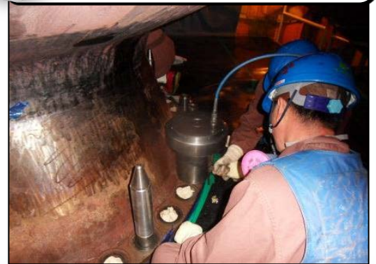
12 Disconnection of S/G lower fixture
