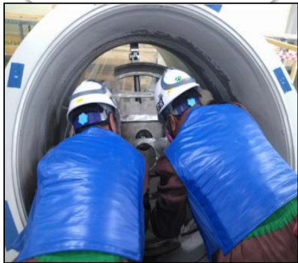
Shielding Plug installation
