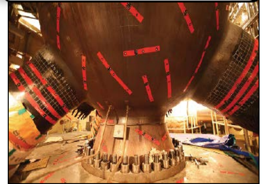
9 Marking the cutting area of RCS pipes
