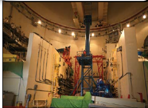
11 Installation of the lifting equipment (TLD/HLU)
