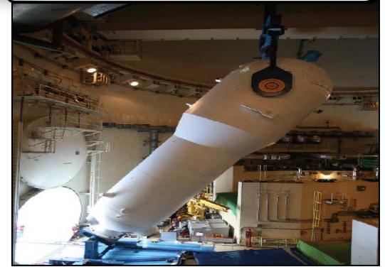
15 Preparation of taking out S/G from RCB
