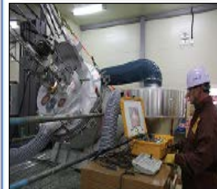
RCS pipes decontamination
