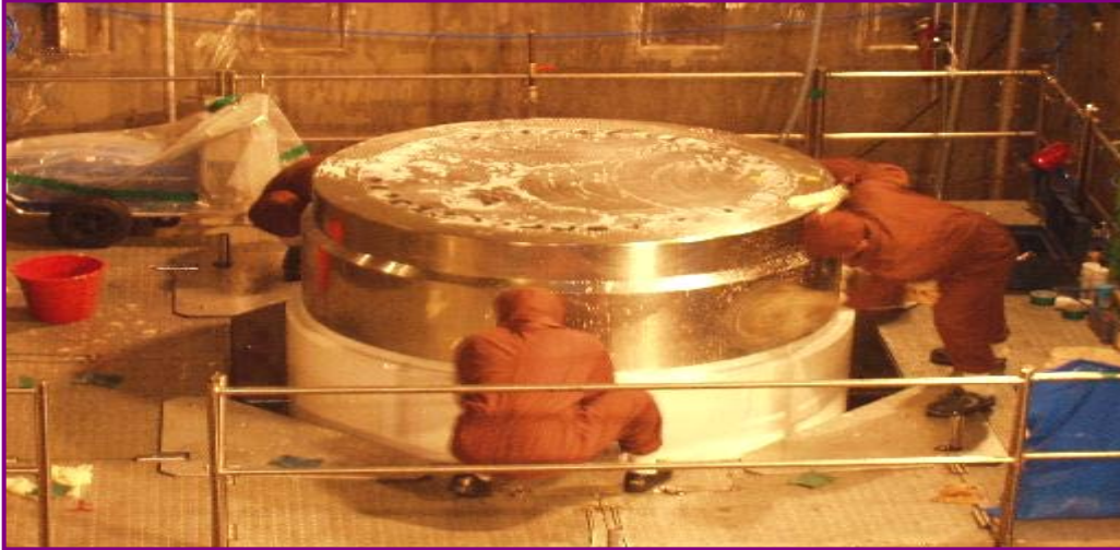
Decontaminating of cask
